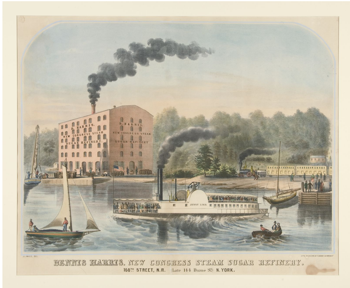
Dennis Harris' New Congress Sugar Refinery on the Hudson River at 160 th Street, with the "Jenny Lind" in foreground, circa 1853. (Yale University Art Gallery)
