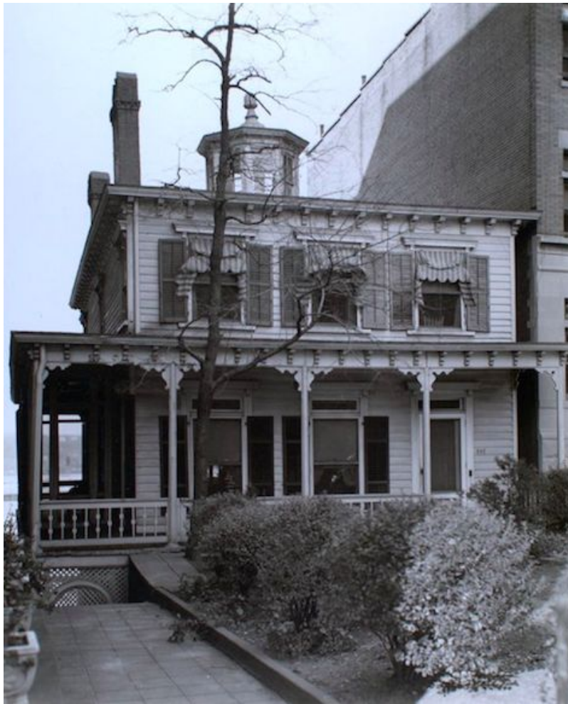
Berenice Abbott photo, taken in 1937, revealing what was at the time a relatively new townhouse next door (859 Riverside Drive), and the house's former river view (seen through the side porch).
