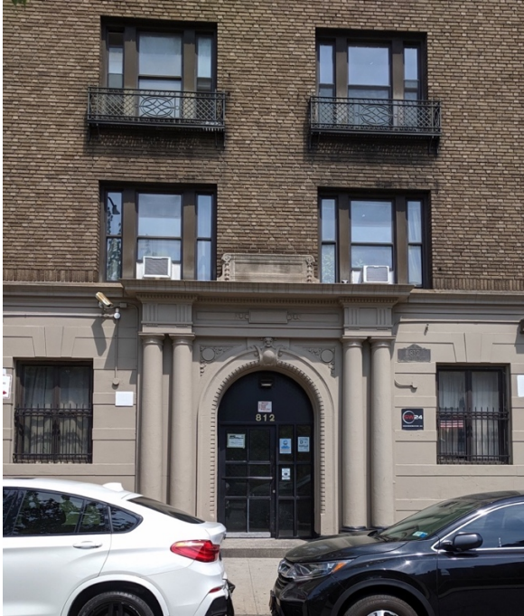
Figure 48: 812 Riverside Drive (Seco Hall)
