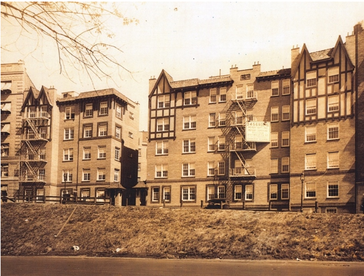
Figure 14: Marion Gardens, 820 Riverside Drive 59
