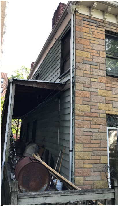
Figure 4 South façade detail showing original clapboard covered in siding.
