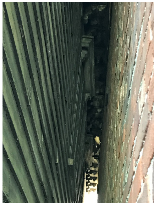
Figure 2 North façade showing preserved window surrounds, shutters and clapboard
