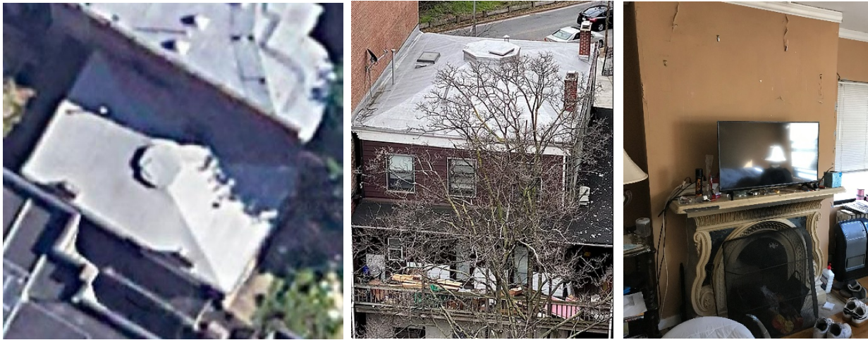
Figures 8-10: Aerial views of the roof and chimneys with corresponding chimney stack and fireplace on the interior
