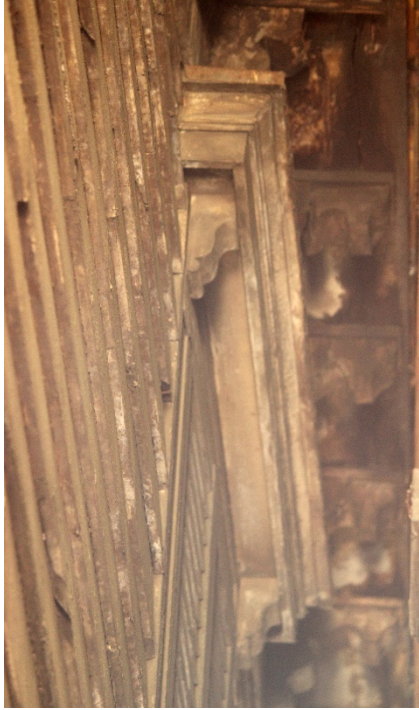
Figure 3 Detail of remaining historic window surrounds and roof brackets, north façade.
